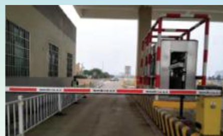
Expressway toll channel
